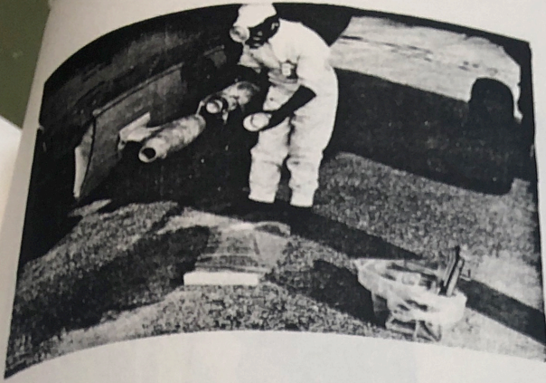
Figure 4(a). Filter Removal. Mk. 8 duct.
